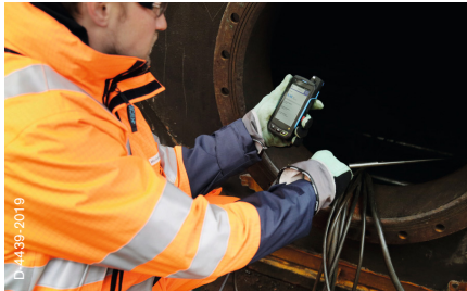
Entry into confined spaces/clearance measuring
