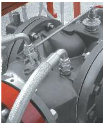
Double Chamber Deluge Valve model VDD
